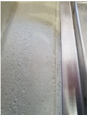
Ensure the drain tray sits flat in the tile tray
